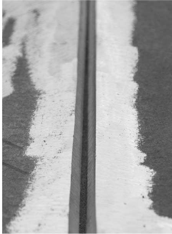
Typical fit-up using a 60 degree Single V-groove.
